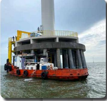
**3.** Manufacturing and installing steel structures for turbine footing (reinforced clamps for pile caps, pillars, supporting structures, handrails, stairs, force platform, monitoring instruments, etc.)
